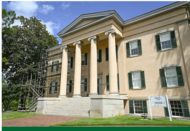
Georgia's Old Governor's Mansion with scaffolding erected ahead of conservation work.
